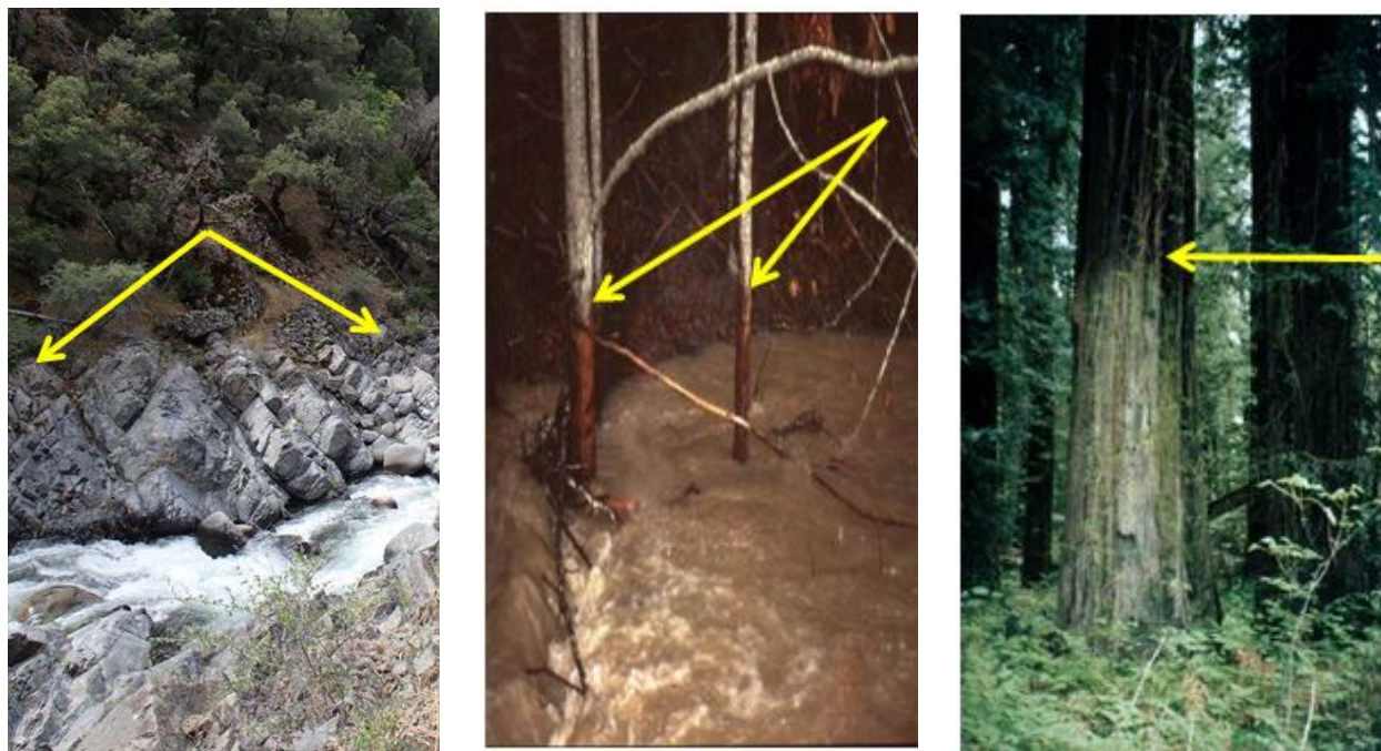
Photo 5.24 - Scour Line (left), Bark Scar (center), and Silt Line (right)
