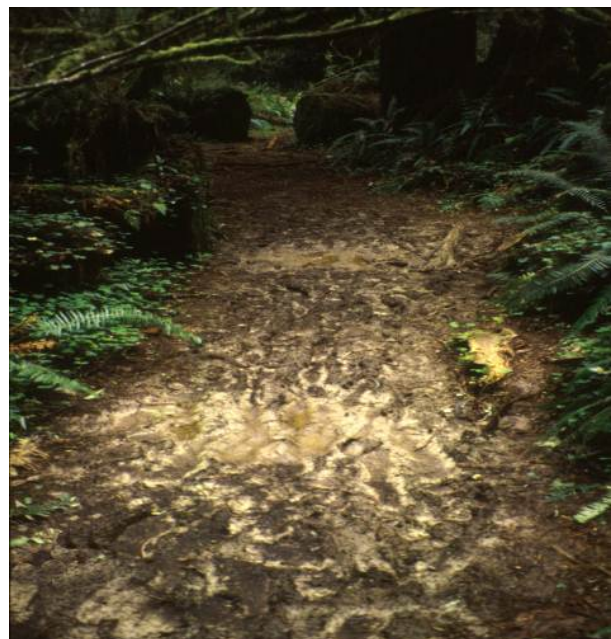
Photo 5.33 - Entrenched Trail (left) and a Saturated and Deformed Trail Bed (right)
