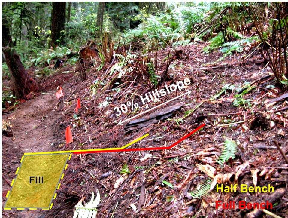
Photo 5.40 - Half Full Bench (yellow line) and Full Bench (red line)
