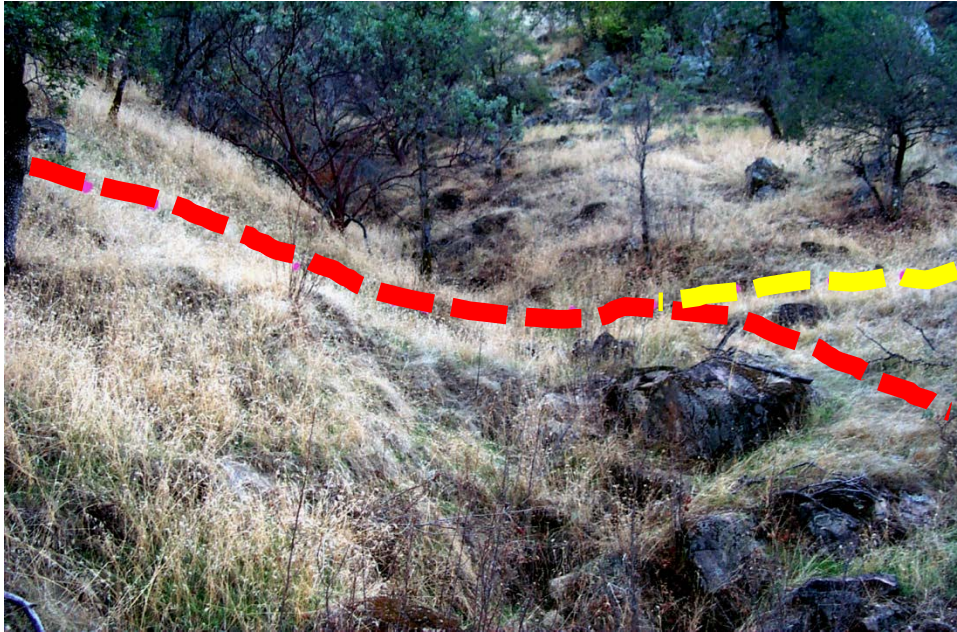
Photo 5.27 - Trail Alignment In and Out of the Influence of an Inner Gorge
