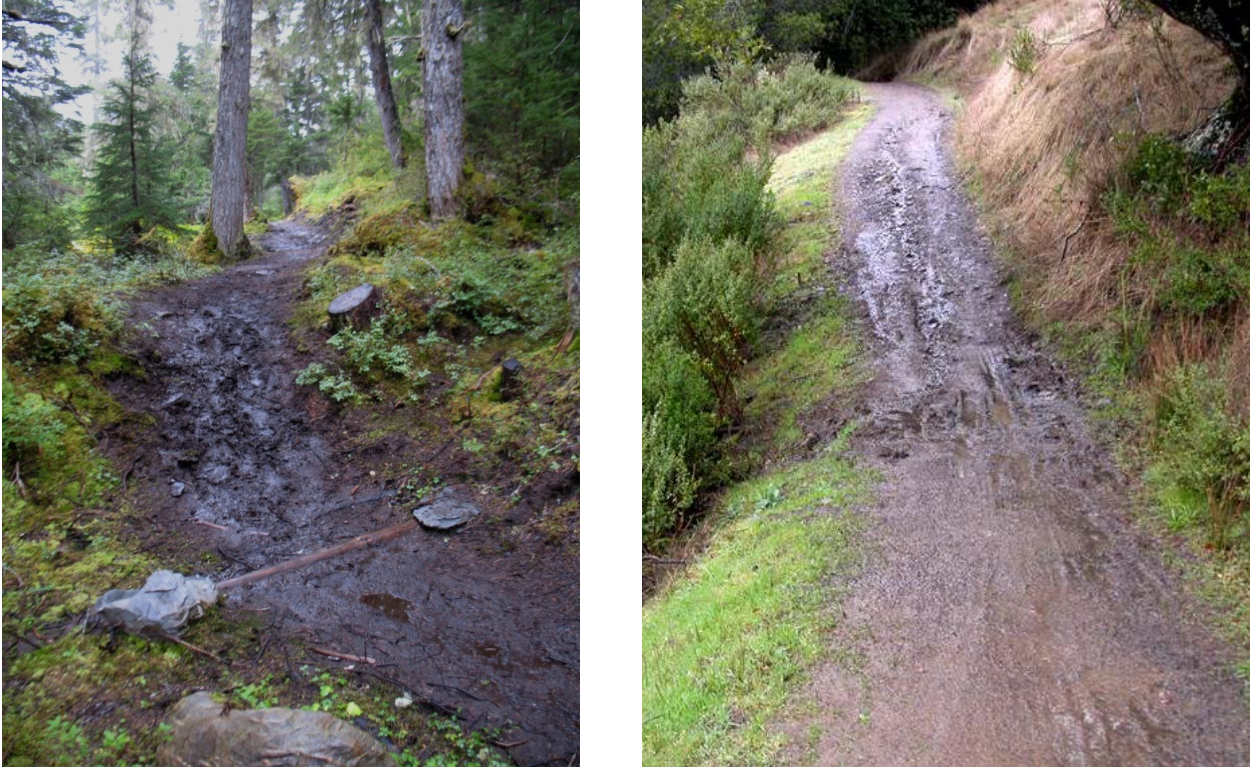
Photo 5.10 - Sudden Grade Increase and Corresponding Mechanical Wear
